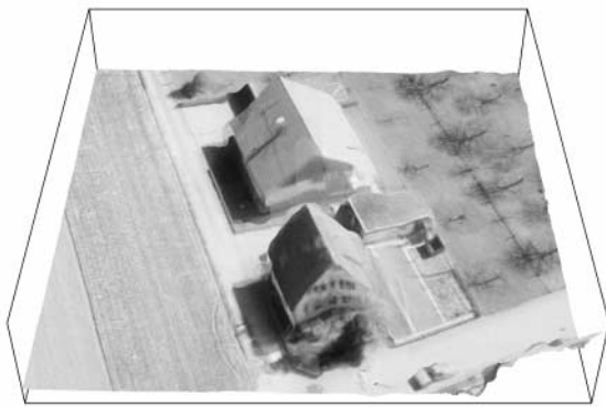
(a) View from west
